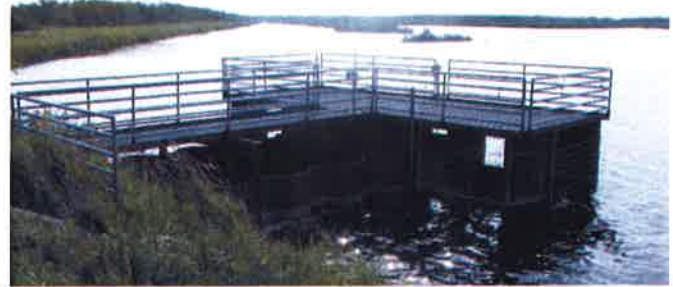
Main Outlet Structure at Nereson Impoundment
