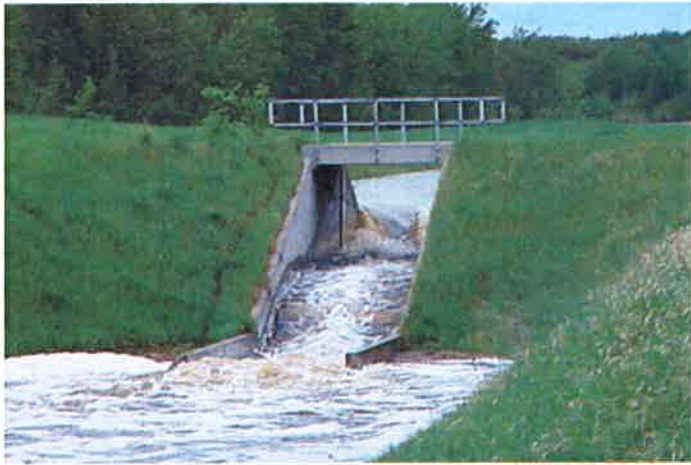
North Branch drop structure – SD 84
