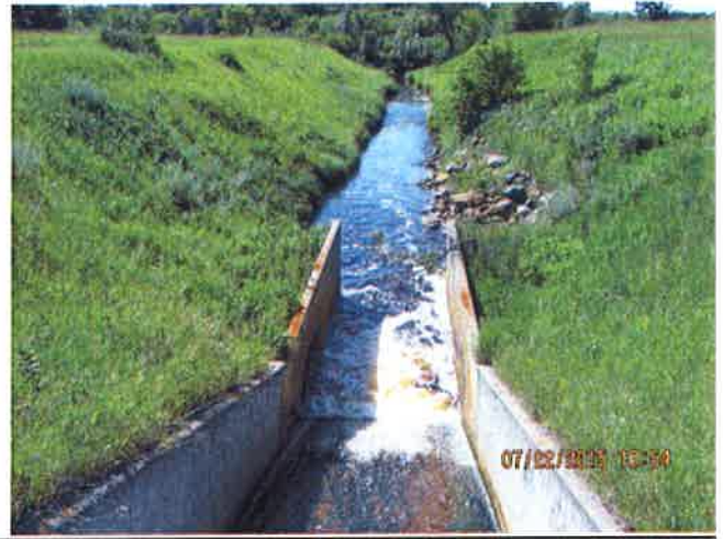
North Branch Drop Structure
