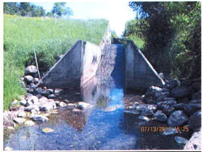
North Branch Drop Structure – JD 31
